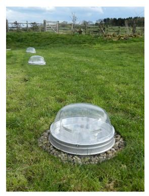
Solarspot D-38 systems pipe light though 500mm of soil and a 300mm thick concrete deck into the 20 metre living space below. RIR light-capture lenses capture direct sunlight and pipe it down into the north-facing room below.
