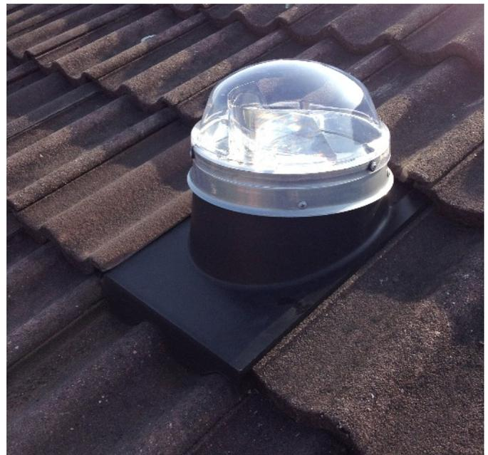
The flashing skirt needs to be cut to the same profile as the tiles it is sitting on (profiled or flat). Using a tile as a template, mark the profile of the lower roof tile onto the front skirt of the flashing.
