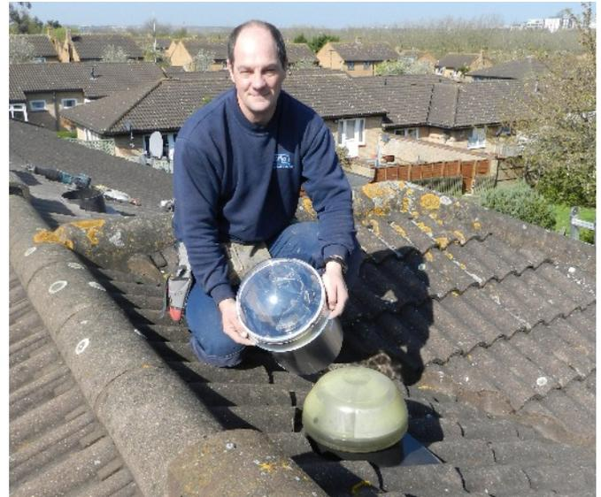
Photo above shows an installer fitting a Solarspot D-25 in a roof where the neighbour has an existing Solatube 160 DS roughly 4 years old. The deterioration of the Solatube dome reduced the levels of daylight down to around 25% of the D-25 unit.
